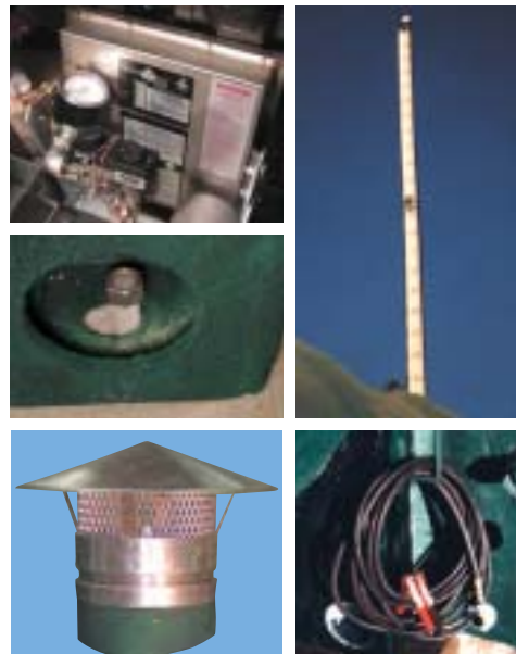
Additional features include; concrete pad with bolts in place, calibrated mechanical liquid level gauge, battery cables, ground wire and screened vents.
