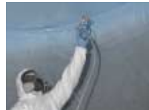
Fabric panels are saturated with resin, curing to create an interstitial space.
