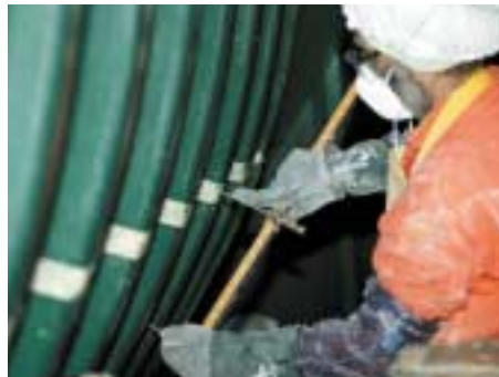
Tank Production, Edmonton
